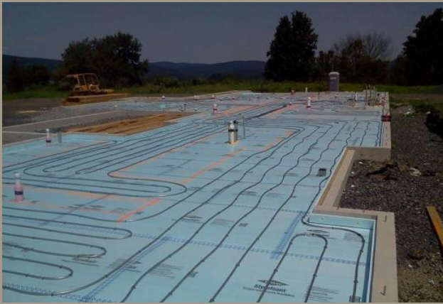
Solar thermal radiant flooring for local calf barn.
